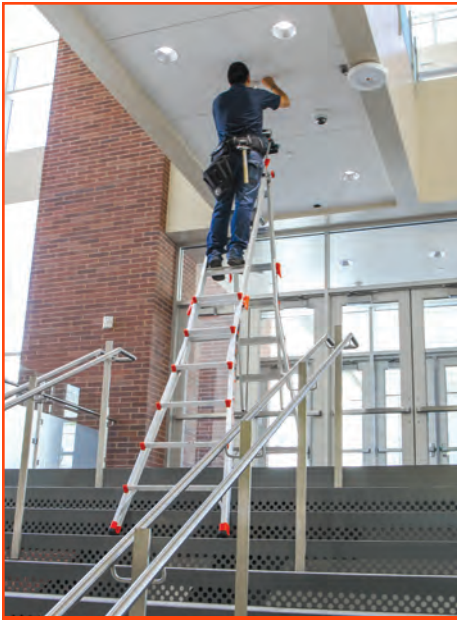
Work over uneven surfaces safely
