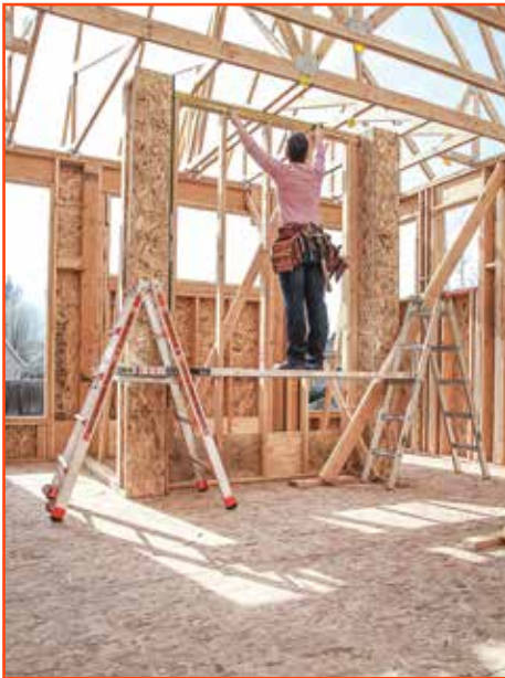
Expand your work area with time-saving scaffolding.
